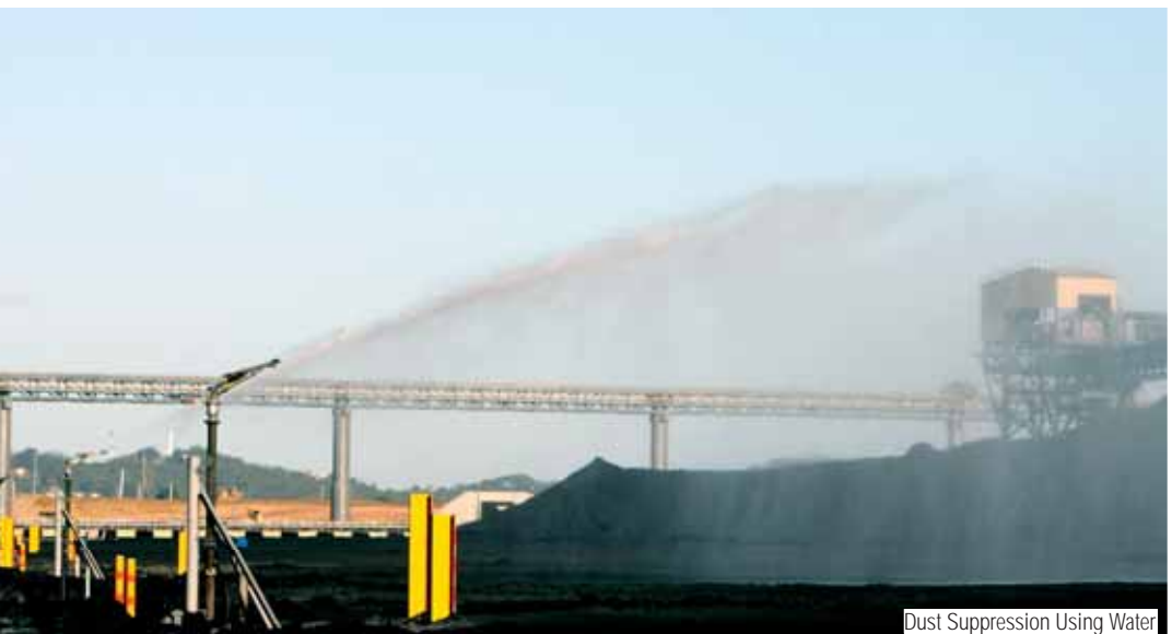
Dust Suppression Using Water
